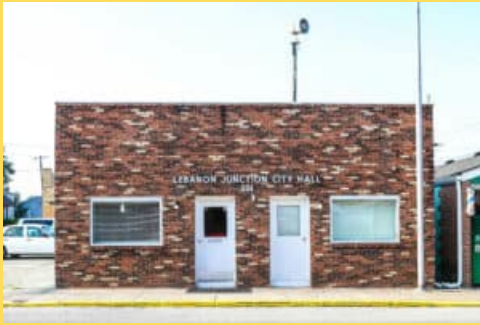
City Hall – 271 Main St
