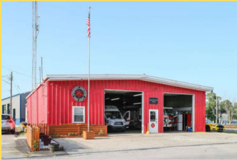
Fire Department – 291 Main St
